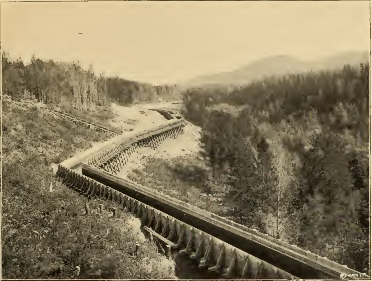
CONSOLIDATED CARIBOO HYDRAULIC MINING CO.'S FLUME.
